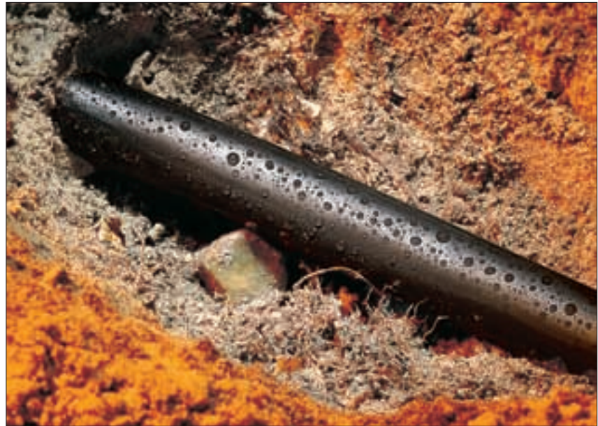
TREDUX HA47 - application below ground.
